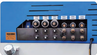
Hydraulic system testing
