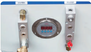
Quick water pressure testing
